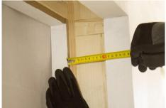
Measure the pocket size at each end and the center where a box will be mounted.
